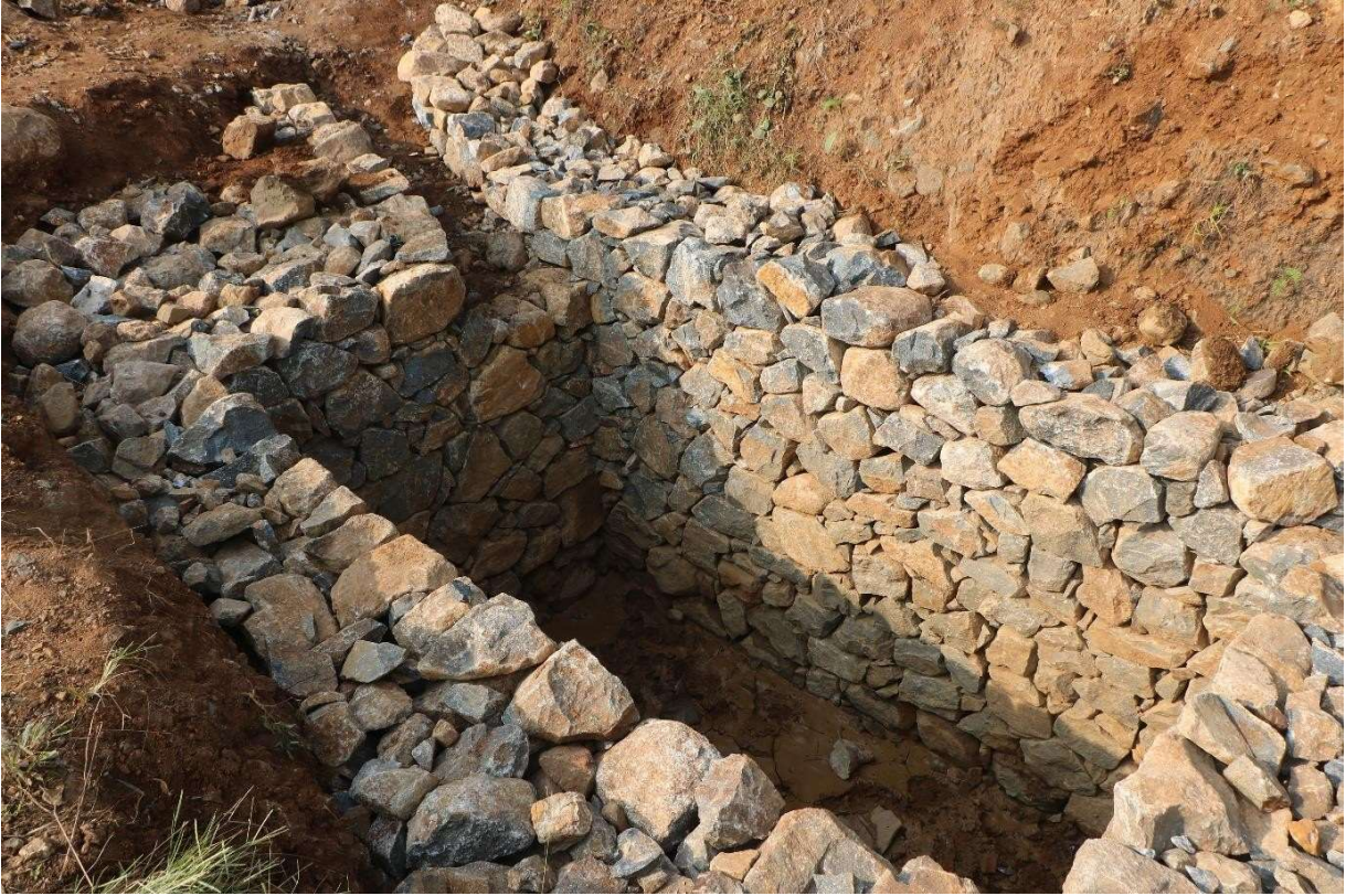
Settling tank for the overflowing water
